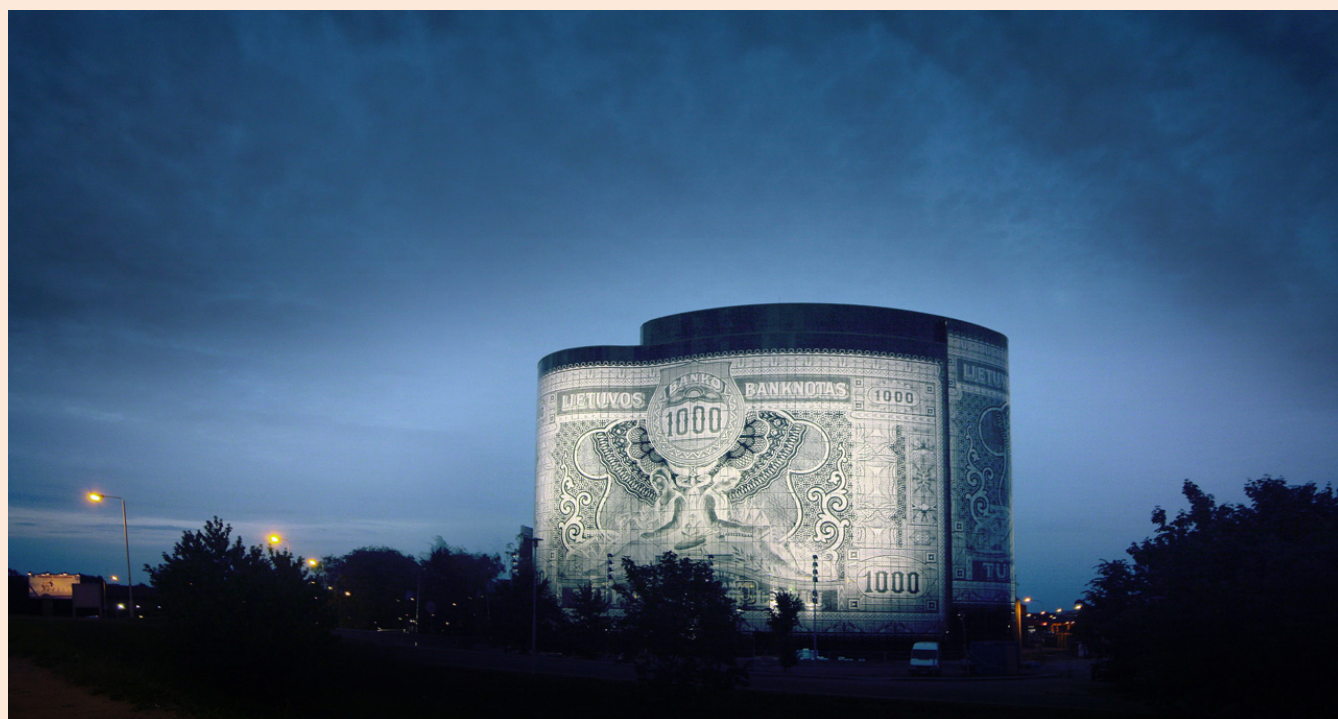
Office center 1000 a.k.a. Banknote Building (Каунас, Литва)
