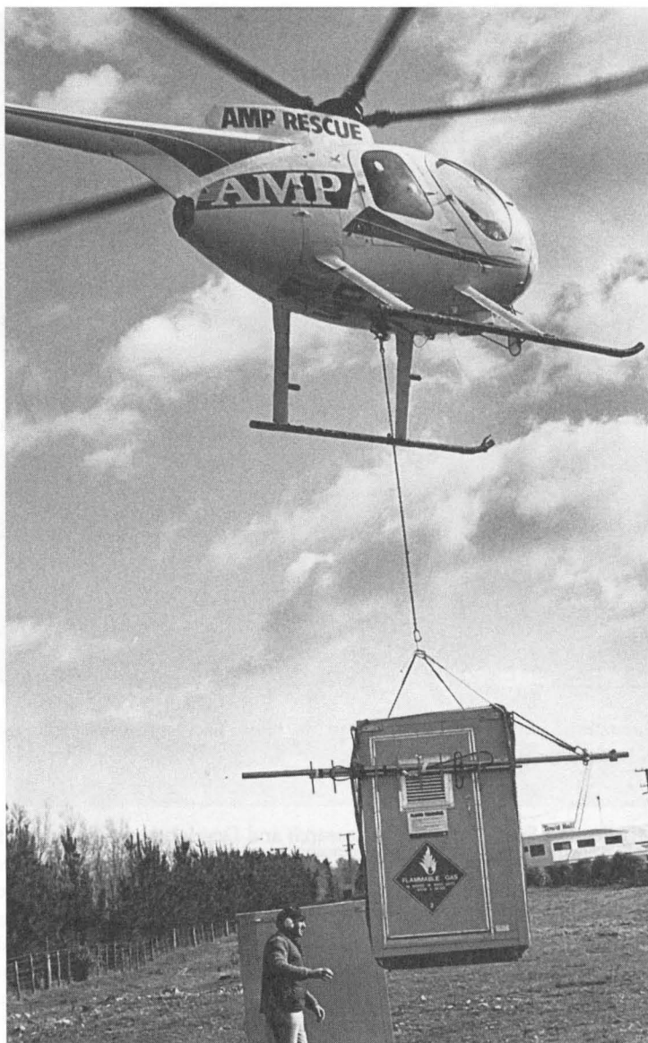
FIGURE 4 Installation of TEG-powered self-contained rainfall data logging and broadcasting system, New Zealand. (Published in the Levin (NZ) Chronicle, 1991.)
