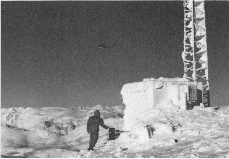
FIGURE 10 Mountain top telecommunications site powered and heated by a TEG.
