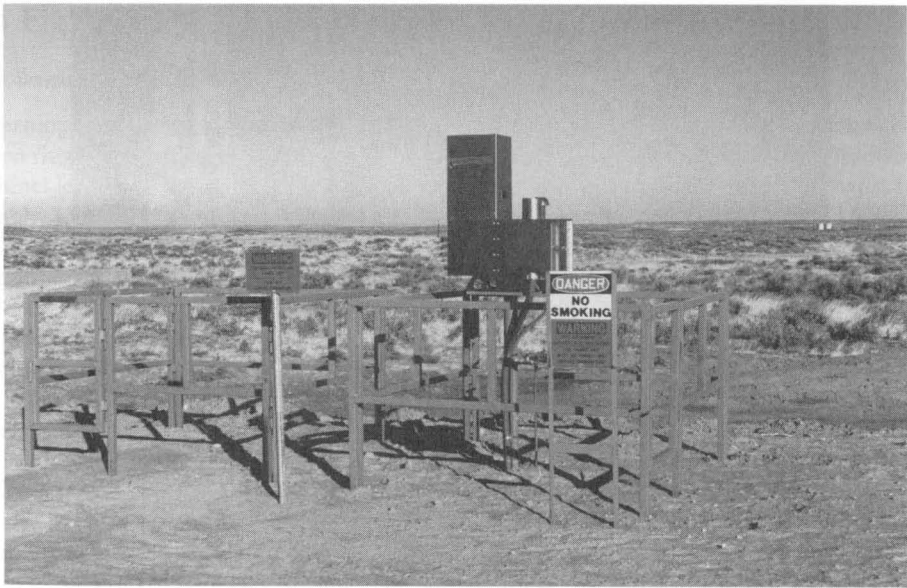
FIGURE 8 120-W TEG used in cathodic protection in New Mexico.
