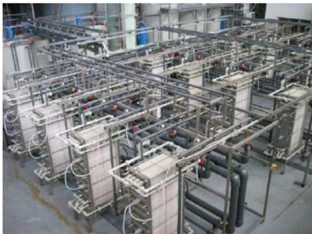
Figure 3.39 EDR modules. Source: MemBrain-MEGA.
