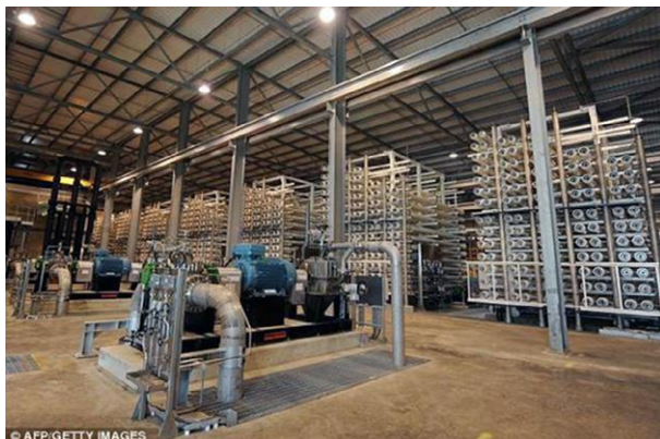
Figure 5.5 Photograph of the 150,000 m 3 /day Thames River seawater-brackish water RO desalination plant. Source: [45].
