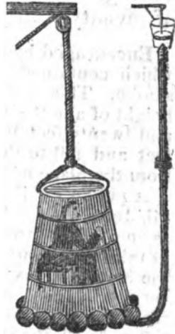
contrivances have been used for diving to small depths, which have answered very well, such as strong cases for the body, to keep off the pressure of the water, which were supplied with fresh air by pipes from the surface. A very good one of this kind is particularly described in the *Philosophical Magazine*, vol. viii. p. 59.
