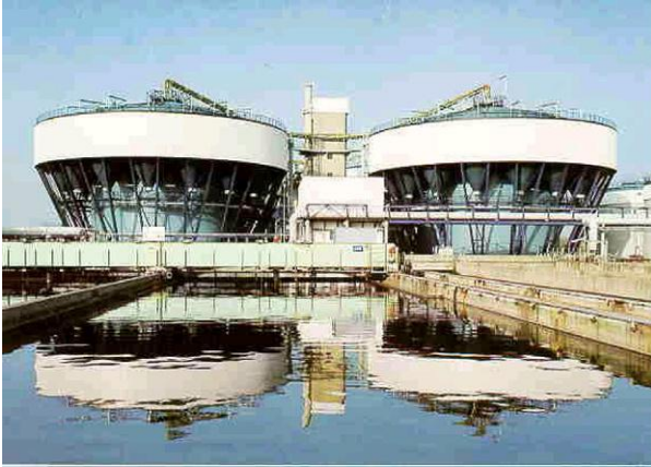
Figure 5.12 Tower Biology at Bayer Leverkusen site.
