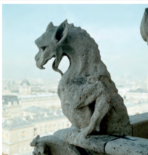
A gargoyle on Notre Dame Cathedral, Paris, photographed in 1996. The damage to the limestone has been caused mainly by acid rain. © Paul Almasy/CORBIS
