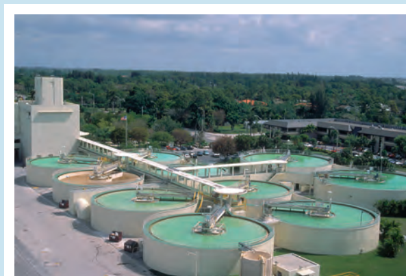
Flocculator-clarifier units in a water treatment plant in Florida, US. Rick Pooley/Visuals Unlimited, Inc
