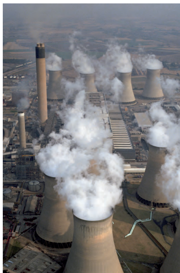
The Drax coal-fired power station in the UK uses desulfurization systems, installed between 1993 and 1996.
