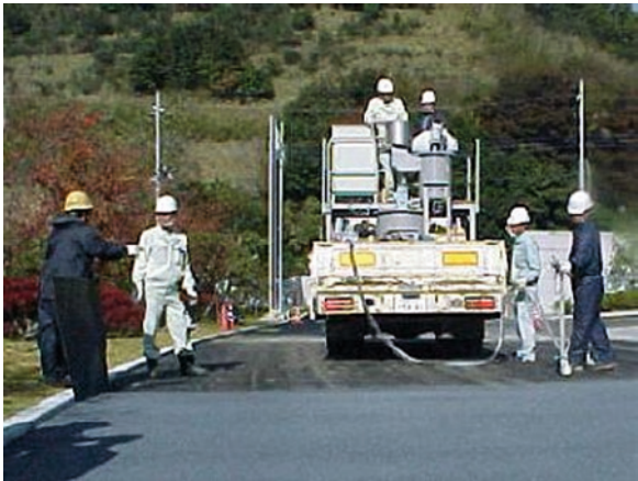
Fig. 5.14 Coating equipment with a mixer and spray applicator for polymer-modified pastes or slurries on a truck (Courtesy of Taiheiyo Cement Corporation)
