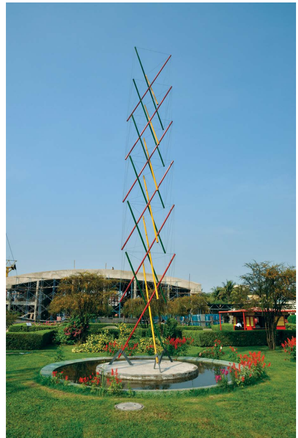
FIGURE 5-31: Tensegrity structure—Science Park, Science City, Kolkata PUBLIC DOMAIN; ORIGINAL PHOTO BY BISWARUP GANGULY.
