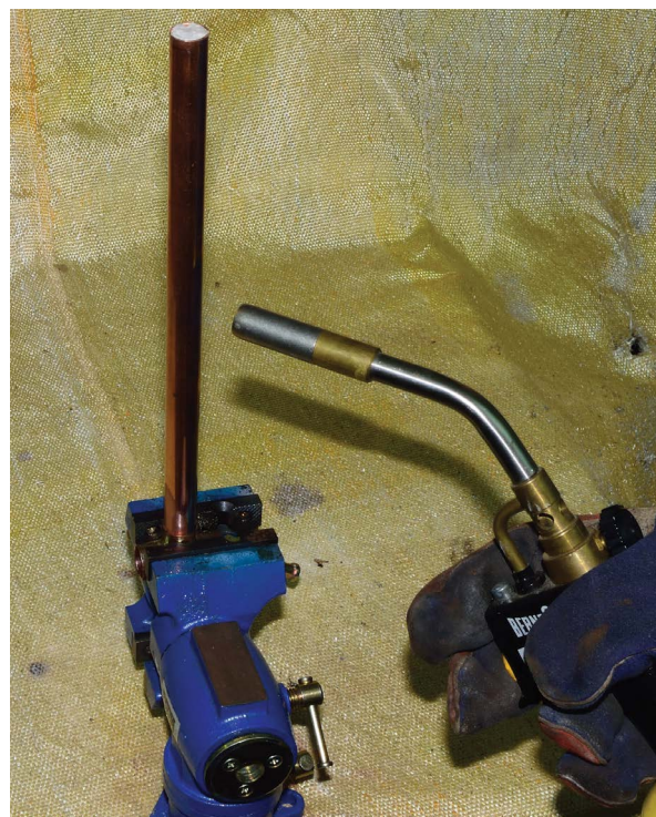
FIGURE 5-12: Heat the tube.
