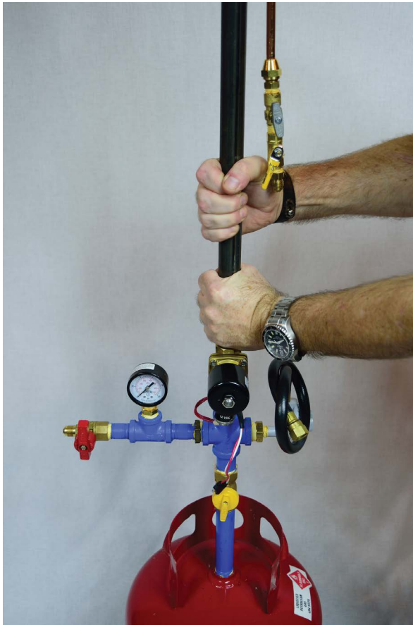
FIGURE 9-33: Attach the main effect pipe.
