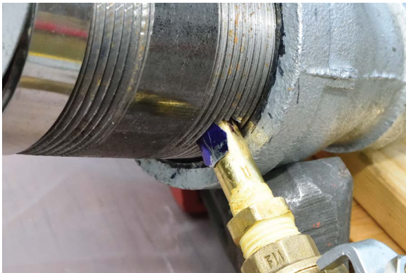
FIGURE 8-19: Shims under the tube
