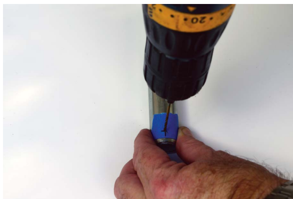
FIGURE 5-33: Drill a pilot hole.
