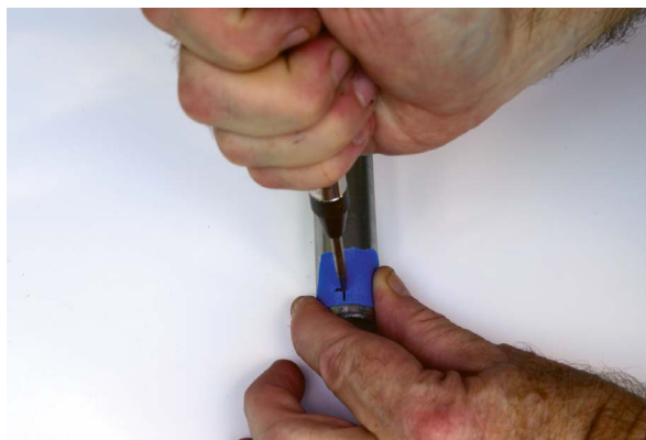
FIGURE 5-32: Mark the hole location on the EMT.
