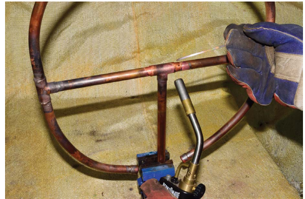
FIGURE 5-22: Braze the side arms into the feeder tee.
