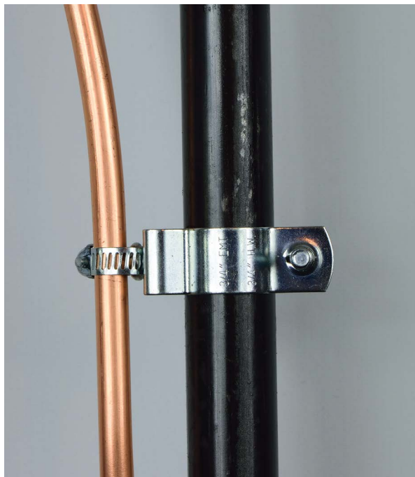
FIGURE 9-32: Attach the pilot to the main effect pipe.
