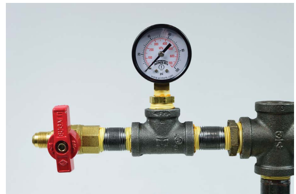
FIGURE 9-10: Gas inlet branch
