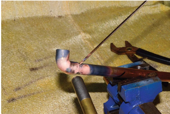
FIGURE 5-20: The 90° elbow faces downward
