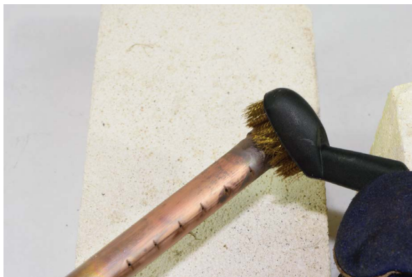
FIGURE 4-20: Cleaning the joint
