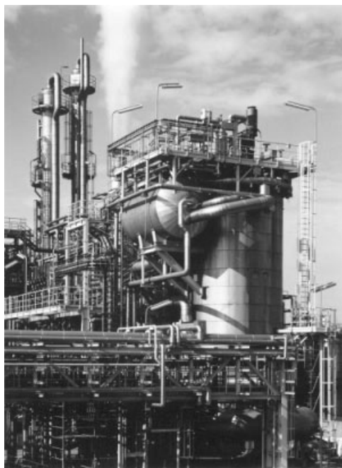
Figure 12.16 Large-scale oxo plant using the water-soluble RCH/RP catalyst \text{HRh}(\text{CO})(\text{TPPTS})_3 . (Note the horizontal decanter in front of the reactor.)
