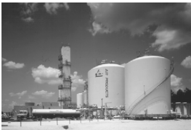
FIGURE 3.48 Flat-bottom storage tanks. (Courtesy of Air Products.)
