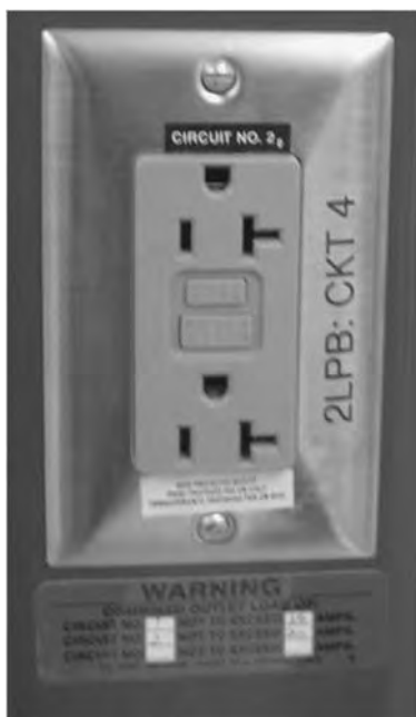
FIGURE 5.3.5.1 Ground Fault Circuit Interrupter (GFCI). These outlets are required at any location near water sources or sinks, although older laboratories may not have these if they have not been upgraded to meet current electrical codes.
