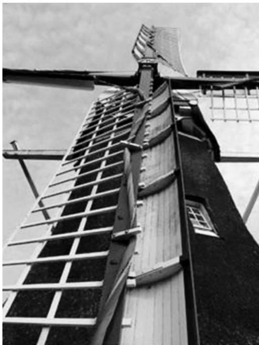
FIGURE 8.14. The blade of a Dutch windmill in Arnhem with the canvas rolled up and secured. See color insert.
