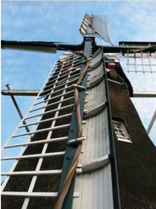
FIGURE 8.14. The blade of a Dutch Windmill in Arnhem with the canvas rolled up and secured.
