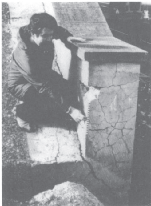
Figure 5.18 Voss Farm Overbridge, Devon, showing a severely cracked wing wall.
