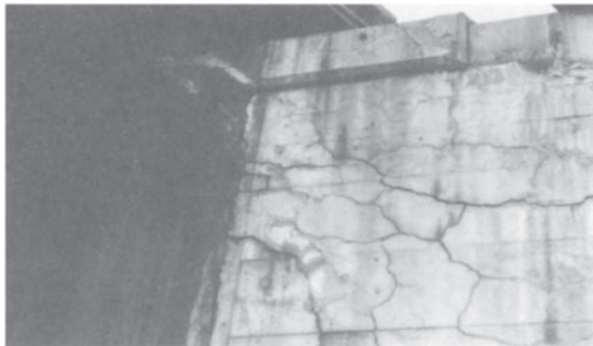
Figure 10.27 Cracking at the corner of an abutment.
