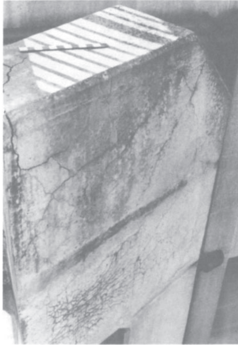
Figure 5.12 Charles Cross Car Park, Plymouth, showing a severely cracked column head.
