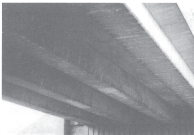
Figure 5.20 Smorrall Lane Overbridge, Warwickshire, showing regular tensile-style cracking of deck beams across the eastbound carriageway. From Ref. 71.
