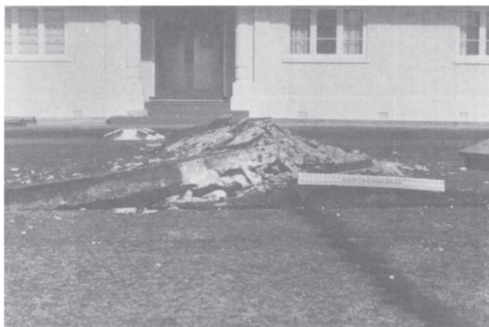
Figure 9.6 This spectacular case of damage occurred in an airbase pavement when 20 years after construction some new concrete was laid abutting one end. The results of restraining the expansion due to AAR were released rapidly during one night.
