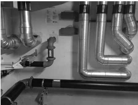
FIGURE 18.2 Inlet pipe in DN150 standard from the Knowledge Center. The bottom pipe was replaced April 2018 due to corrosion. The pipe had been in operation for five years.
