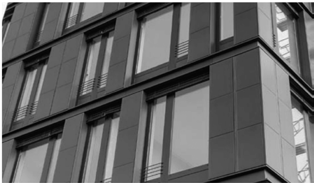
FIGURE 14.5 CIGS modules as facade elements on the ZSW building in Stuttgart, Germany.
