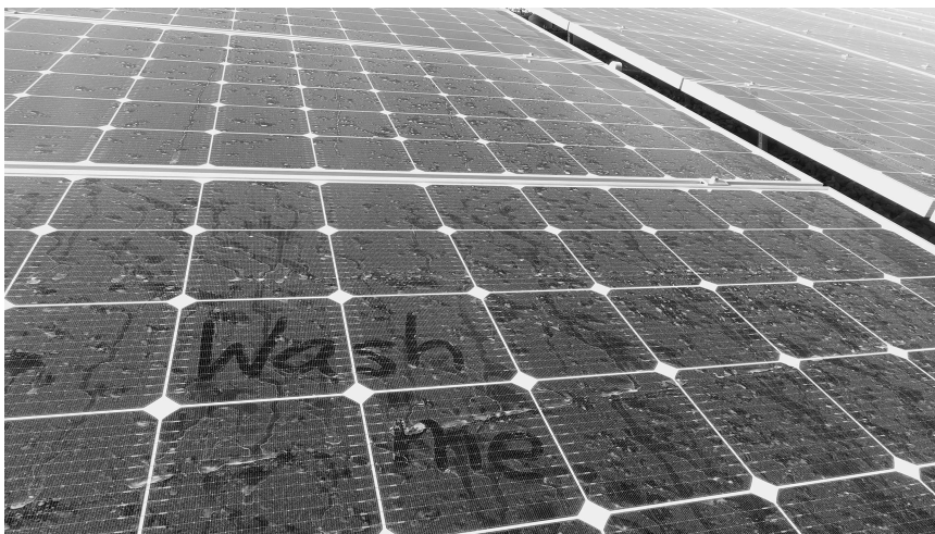
FIGURE 17.5 A dusty photovoltaic panel.
