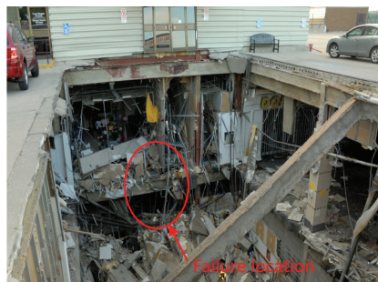
Figure 1.2 Collapse of a parking deck.
