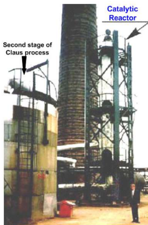
Figure 20. Semi-industrial installation for the direct oxidation of hydrogen sulfide via monolithic catalyst with a honeycomb structure. Tail-gas of the Claus process.
