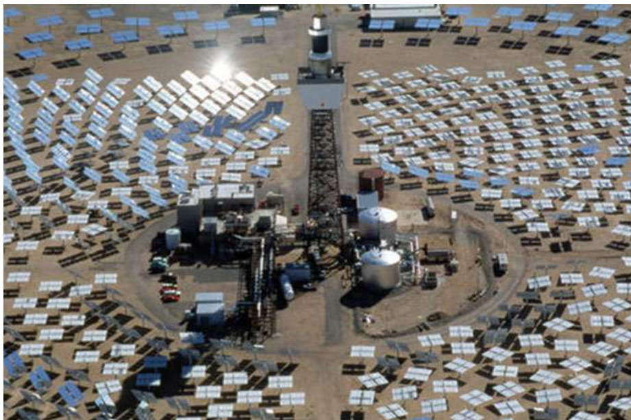
Figure 8.4: Solar power tower CSP.
