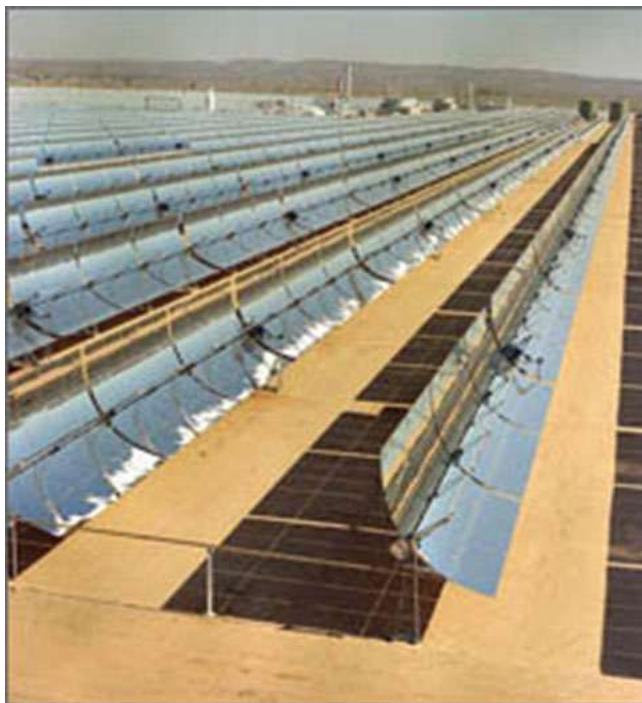
Figure 8.3: Parabolic troughs for CSP.
