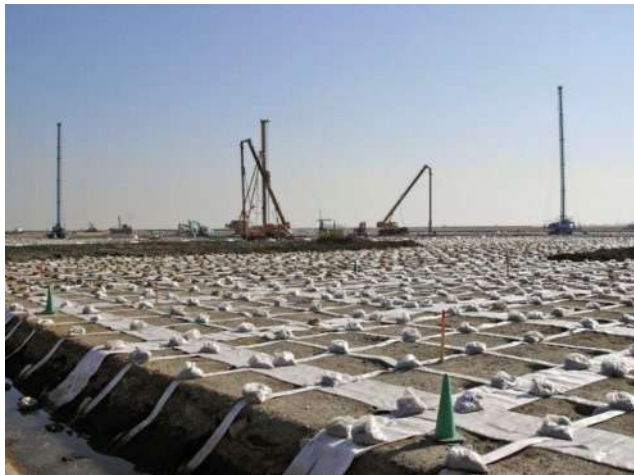
FIGURE 27.13 PLA vertical drain sheets. Source: Chikami Miltec, Inc.
