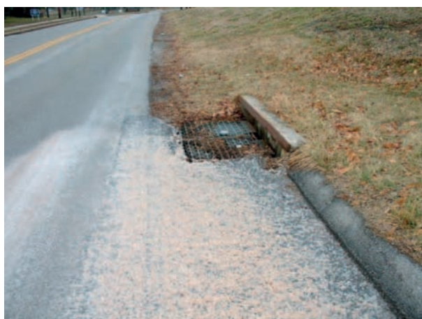
Figure 2 Road salt crystals near a storm drain entering a major drinking water supply in Baltimore, MD, USA. (Photo courtesy of Ken Belt.)
